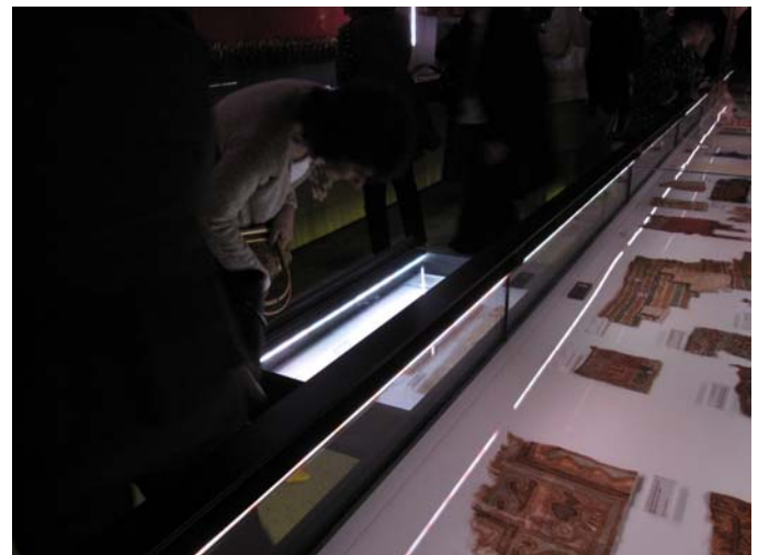
Motion-activated LED case lighting (including drawer lights) and downlighting provide all light for the textile gallery at Museo Chileno de Arte Precolombino
